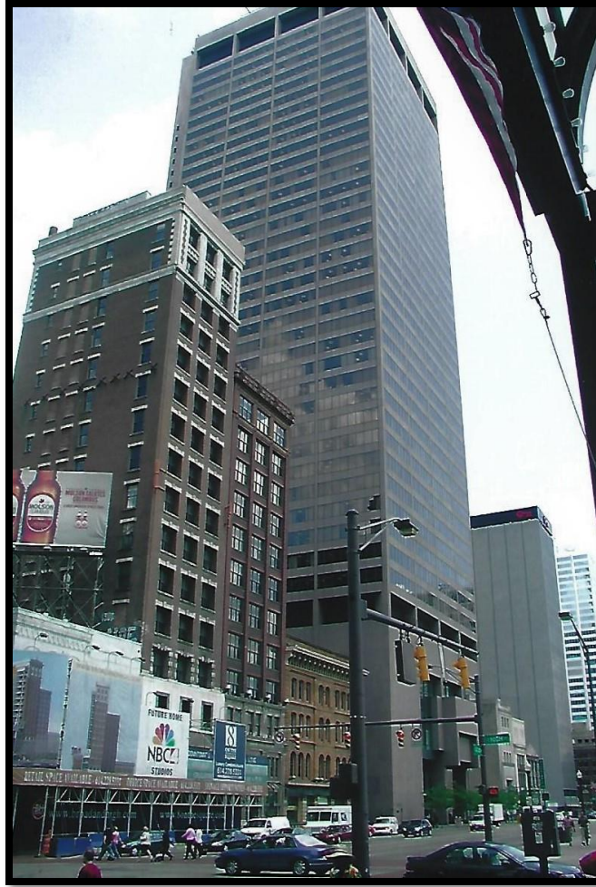
Photo Northeast Corner of Broad and High in 2005
