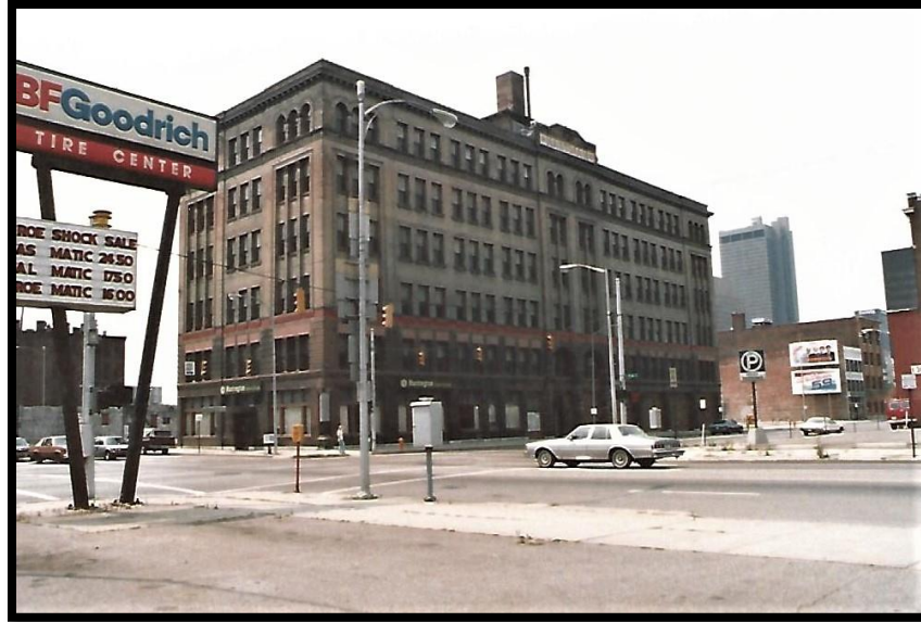
1985 Northwest Corner of Main and Fourth
