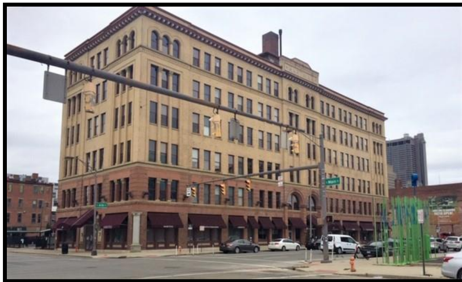
2020 Northwest Corner of Main and Fourth
