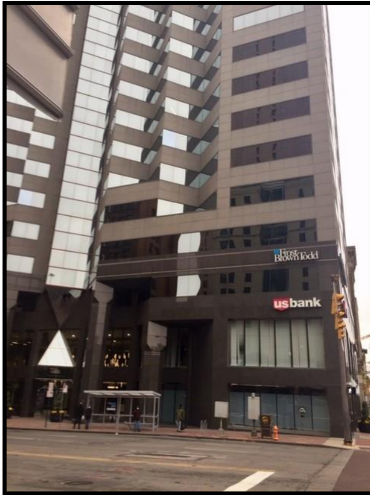
2020 Northwest Corner of Broad and High
