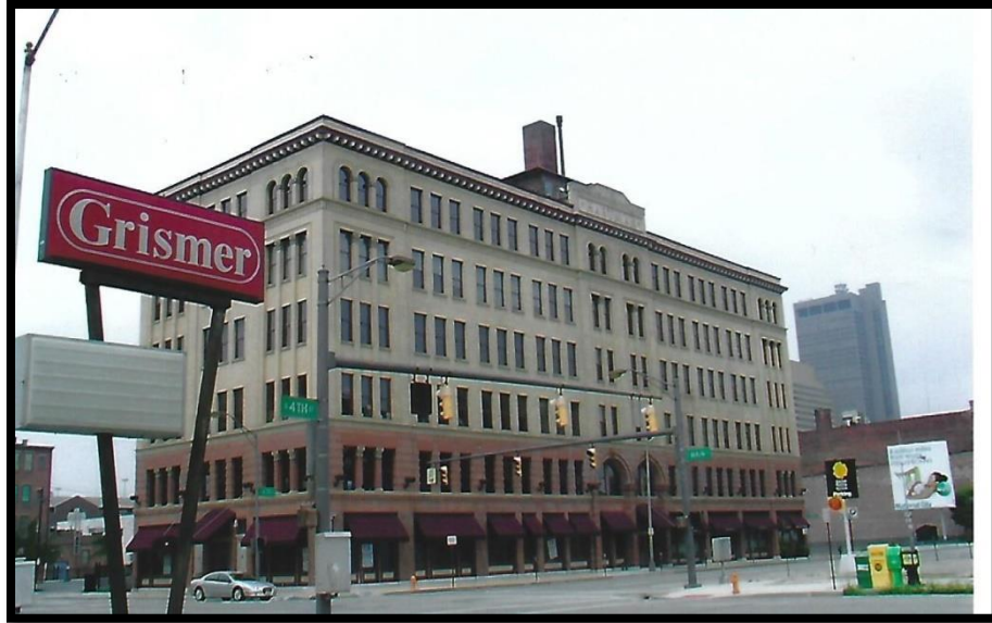
2005 Northwest Corner of Main and Fourth
