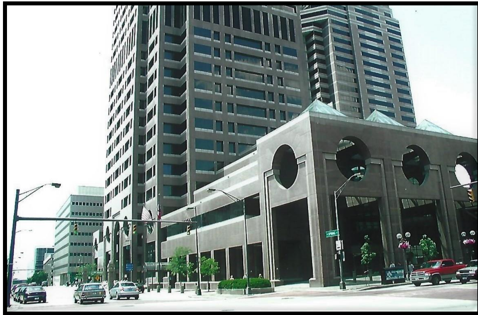
2005 Northwest Corner of Spring and High
