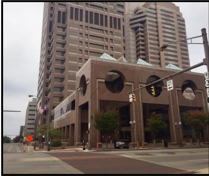
2020 Northwest Corner of Spring and High
